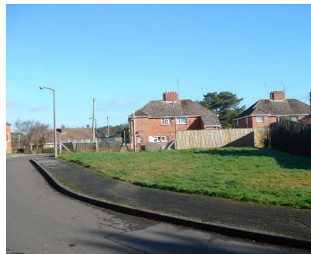
3. Poorly used, left over open space is a feature of Bovington, seen here at Morris Road
