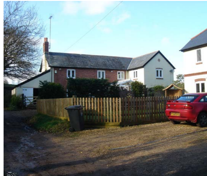
1. Cottages on King George V Road, north of Stanley Barracks are of Critical townscape quality because they maintain a visual and historic association with the wider rural setting.
